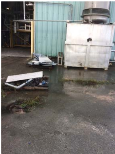
Photograph 1: Activation Process Cooling Tower and Water Discharge
